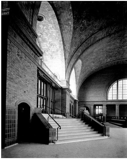
Figure 6: Interior Steps of the Third NY Central Railroad Station
