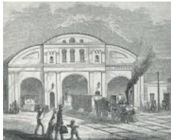
Figure 2: The front of NY Central Station
